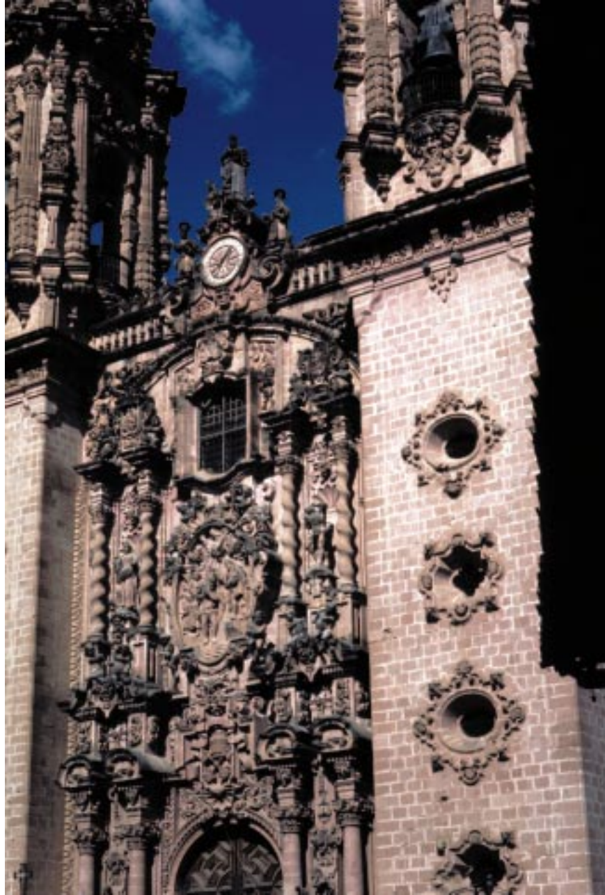
Made of local sandstone, the masonry is as ornate and well crafted as any found in Europe
