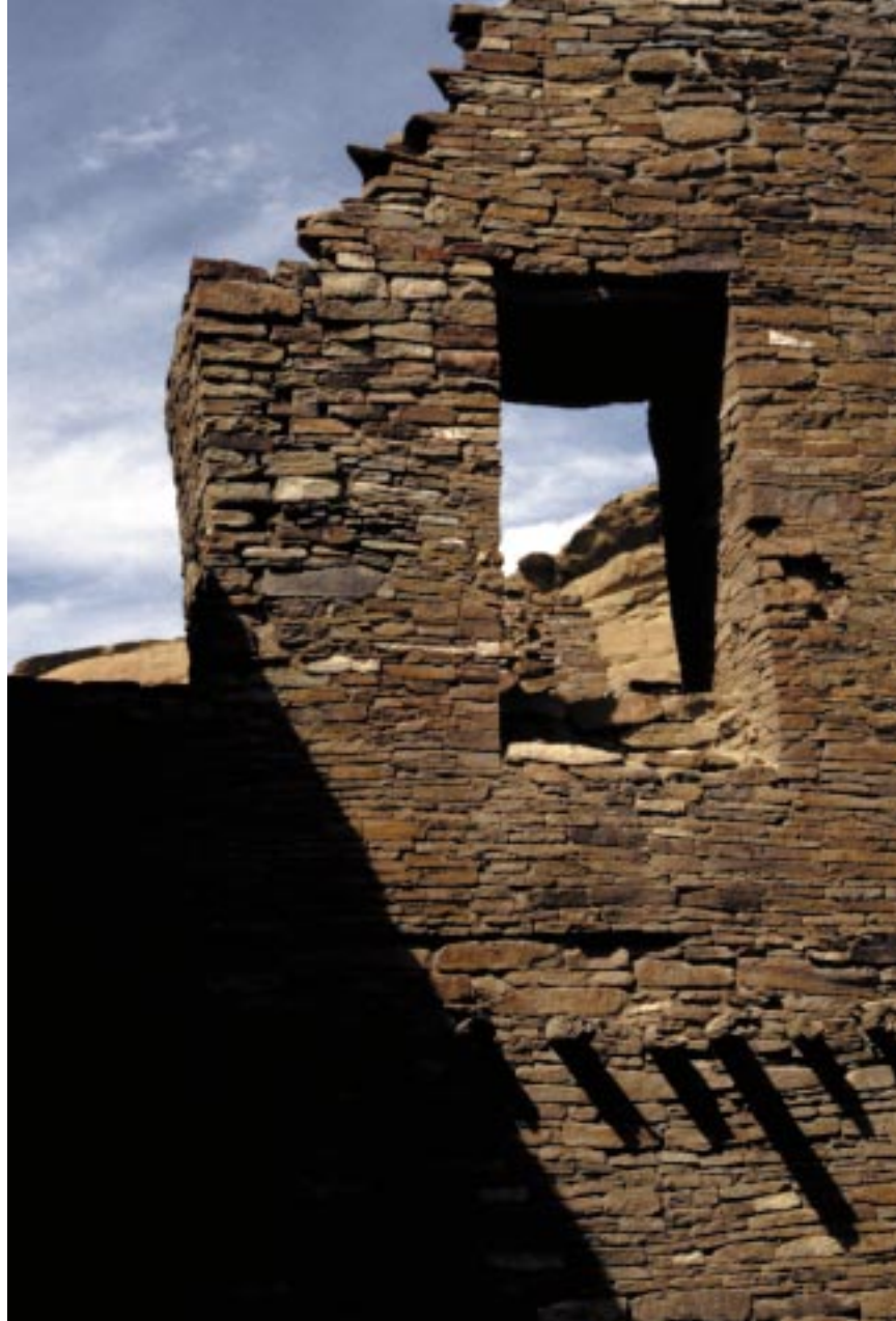
A view into the past. The exquisite masonry easily rivals anything constructed by the robber barons of Europe during the middle ages.
